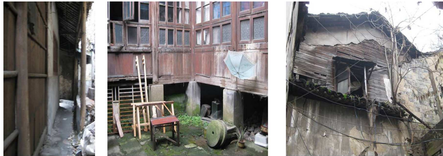
Figure 3 Photos of the case historic residential building
